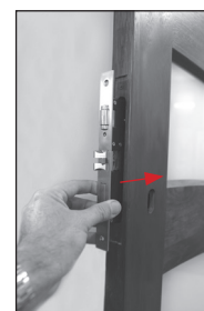
INSERT AND FIX LATCH TO DOOR
