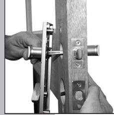
Insert the spindle through the Latch then place the external trim plate against the door. The bottom tail piece MUST BE in the horizontal position and pass through the Deadbolt '+' section. Then place the internal trim plate into position.
