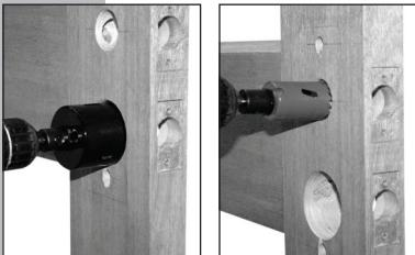
Drill all holes in the door face remembering not to drill all the way through the door from one side. Drill from both sides to avoid splintering.
