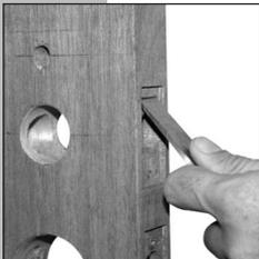
Chisel out the timber to a depth of around 3mm deep to allow the Latch and Deadbolt to sit in flush with the door edge.
