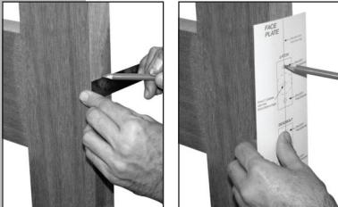
Next, mark the centre of the door edge. Using the face plate template, align the centre of the template with the centre line on the door edge, then mark all hole positions.
