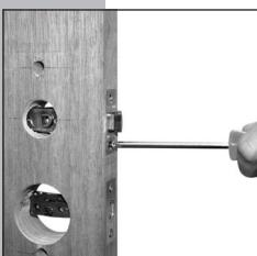
Insert the Latch into the top hole, ensuring the taper on the Latch is positioned towards the door jamb where the strike plate will be located. Place the Deadbolt into the bottom hole, observing the 'up' direction indicated on the Deadbolt, then screw into place with the short wood screws supplied.
