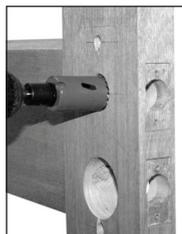
Drill all holes in the door face remembering not to drill all the way through the door from one side. Drill from both sides to avoid splintering.
