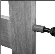
Drill the 25mm (1") holes (x2) in the edge of the door to a depth of around 95mm. (Ensure that these holes are drilled squarely). Insert the Latch in the top hole, Deadbolt in the bottom hole then mark around the face plate ready for Mortising.
