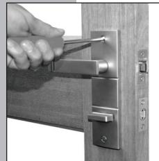
Secure both trim plates with the two long metal thread screws. Tighten the screws and check all locking operations work freely.
