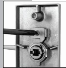
Replace and tighten the screw that holds the lever handing stopping block and the change of handing is now complete. This process is required on both the inside and outside trim plates, if initial preset set handing is not suitable.
