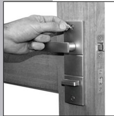
When you are positive that all locking operations work, push in place the screw cover supplied. N.B. There are four screw covers supplied in the event you need to remove the lockset at a later date then re-install.
