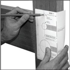
Using the template supplied, mark all locations where you need to drill. For accuracy and alignment, fold the edge of the template where shown around the door edge. The two lines on the template edge that folds around the door will be the position for the Latch and Deadbolt.
